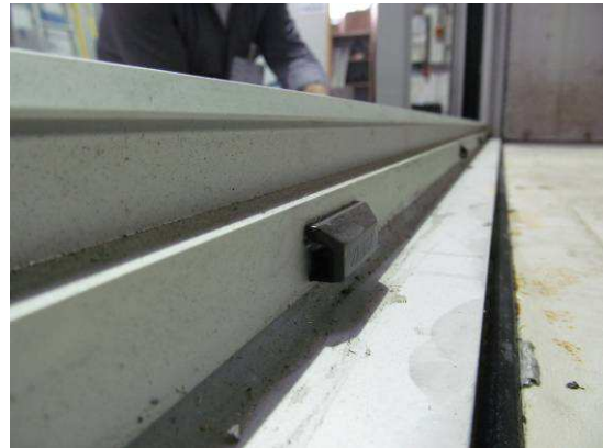
Fig. 7 Drainage external
