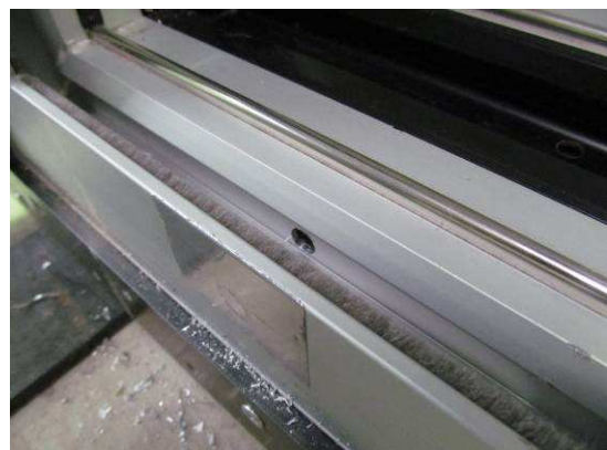
Fig. 11 Drainage drilling for inside channel
