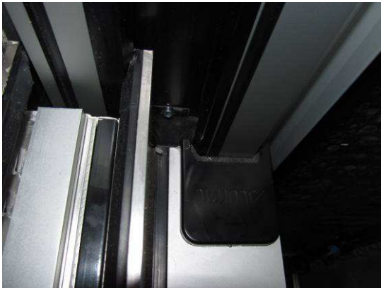
Fig. 6 Central meeting joint seal at top
