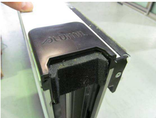
Fig. 4 Central meeting joint at top, corner design
