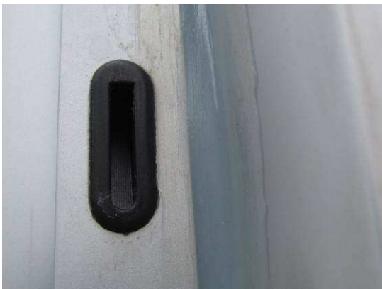
Fig. 8 Pressure equalization frame profile
