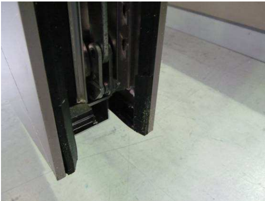
Fig. 2 Casement seal at bottom, corner design
