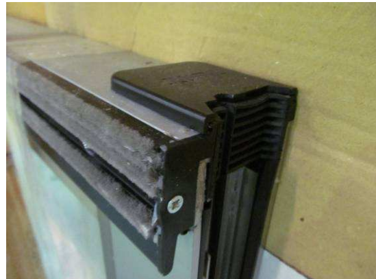
Fig. 3 Central meeting joint profile at bottom, corner design
