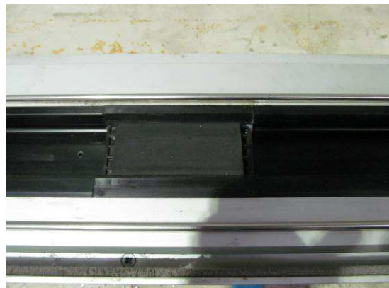
Fig. 5 Central meeting joint seal at bottom
